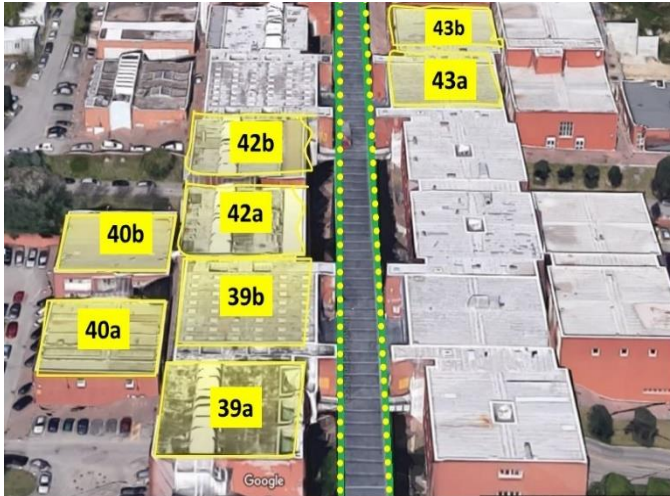
Fig. 13. The Smart UniCal infrastructure: the SmartBridge part (dotted yellow bordered area) which crosses the SmartDIMES (yellow bordered area with building identification codes).
